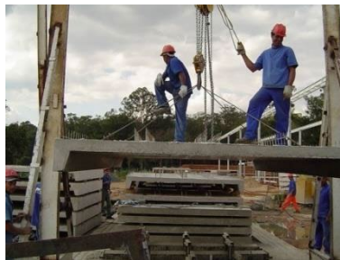
Figure 9: Production of precast concrete slabs Source: personal archive of Fabricio (2005).
