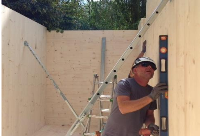
Figure 5: The construction of the load bearing structure with XLam panels
