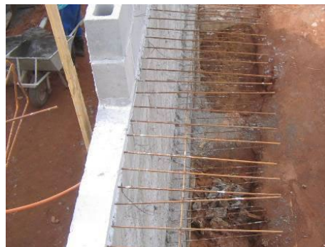
Figure 3: Retaining wall Source: personal archive of Verniz (2009).
