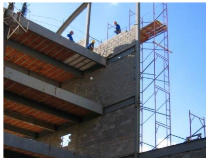
Figure 14: Concrete-block masonry in external walls Source: personal archive of Verniz (2010).
