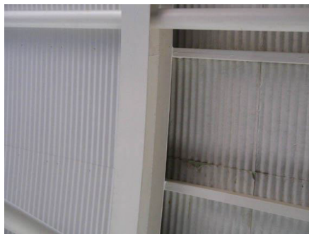
Figure 23: Detail of metallic roofing Source: personal archive of Verniz (2010).
