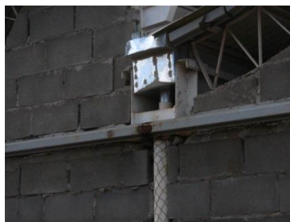
Figure 15: Binding of masonry to column using wire mesh Source: personal archive of Verniz (2010).
