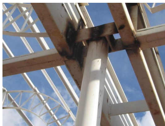
Figure 4: Metal column and beam Source: personal archive of Verniz (2009).
