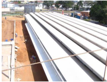
Figure 20: Roof of Services Wing Source: personal archive of Verniz (2011).
