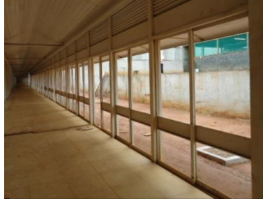
Figure 16: Metallic window frames Source: personal archive of Verniz (2010).
