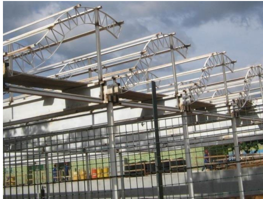
Figure 5: Roof made with metal trusses Source: personal archive of Verniz (2009).
