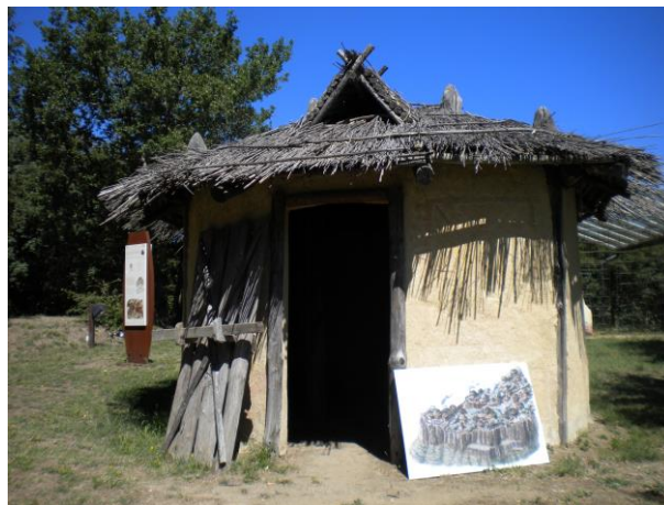
Figure 2: Reconstruction of a proto-historic hut, late Bronze Age, with roof in wooden structure covered by small canes closely tied together (Open air Museum Alberto Manzi in Pitigliano - GR)
