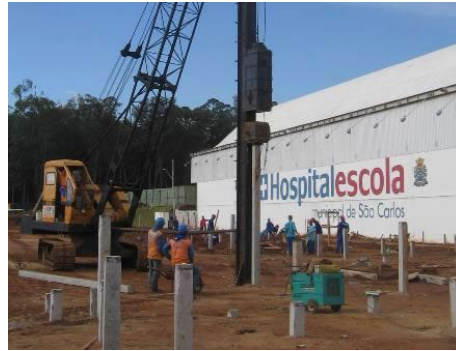
Figure 2: Precast piles Source: personal archive of Verniz (2009).
