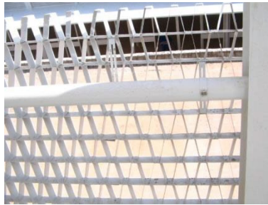
Figure 17: External walls of the Admissions Ward Source: personal archive of Verniz (2010).
